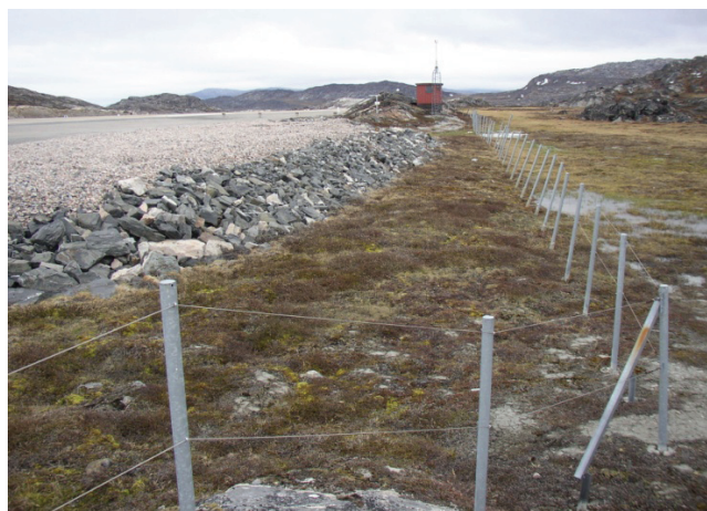
Figure 7. Photo of the tilt and heave of the fence pile due to a horizontal slide of the rock fill slope guided by deformation in the active layer.
