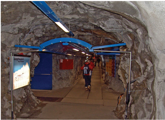
Figure 3. A roof protects tourists from melt water that only recently began to percolate through the rock mass above the tunnel inside the Jungfrauoch rock crest, 3500 m asl, Swiss Alps.
