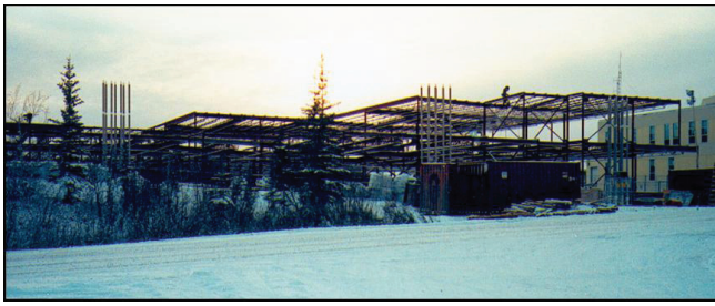
Figure 5. Inuvik Hospital – open foundation and framing stage, October 2001.
