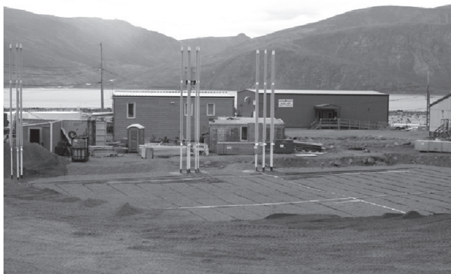
Figure 4. Typical thermosyphon flat loop, slab on ground installation at Pangnirtung, NU.
