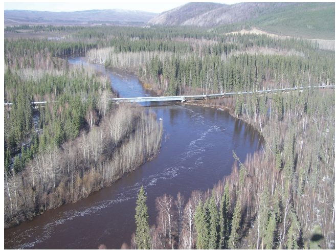
Figure 5. Post-construction spring breakup 2006, as compared with Figure 1. Overbank flow completely submerged floodplain and deflector vanes. No bank erosion, and main flow current is along the tip of deflection vanes, away from the right bank (note location of white “bubble line”).
