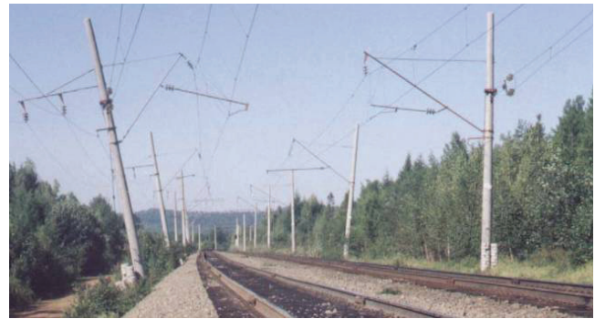
Figure 6. Adverse deformation of power line tower supports along the electrified section of the Transbaikal Railway, August 2001.
