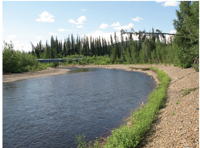
Figure 4. Hess Creek upstream of pipeline bridge. Willows were planted along the bank and on the newly created floodplain.
