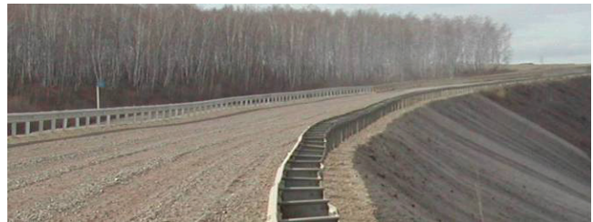
Figure 9. Same section of road on the “Amur”–Chita to Khabarovsk Highway, km 247, one month after completing innovative repairs, October 2006.
