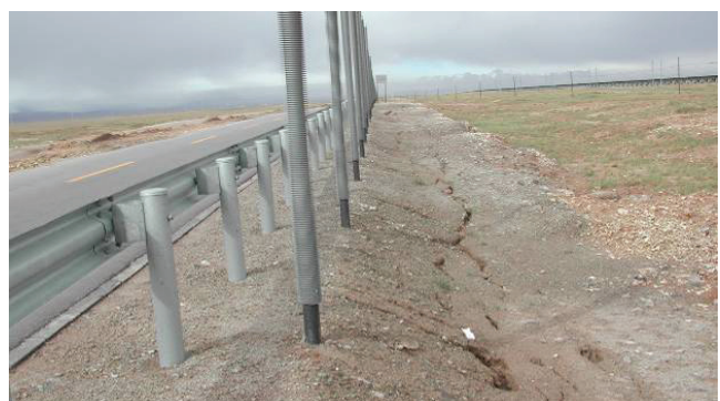
Figure 11. Deformation and displacement of an embankment slope on the Qinghai–Tibet Highway as a result of permafrost degradation outside the influence area of the thermosyphons, August 2006.
