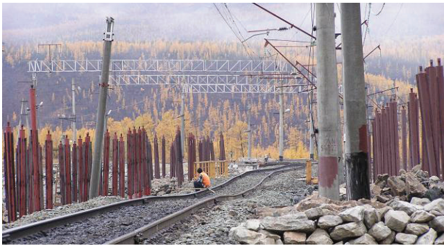
Figure 2. Area of severe deformation on the East Siberian Railroad at 1374 km of BAM, September 2003 (photo by E.A. Kozyreva).
