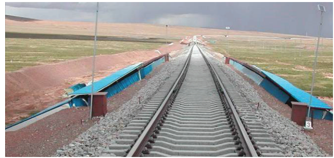
Figure 4. Sun-precipitation protective sheds on the Qinghai–Tibet Railway, August 2006.
