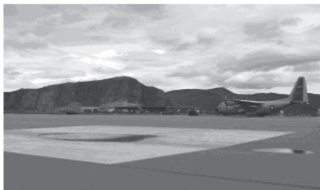
Figure 3A. White painted asphalt surface on the southern parking area of Kangerlussuaq Airport.
