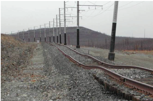
Figure 3. Track and power line tower deformation along the Chara–Cheena Railroad, October 2003.
