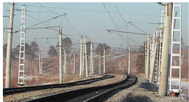
Figure 1. Deformations of a track and power line tower support along an electrified section of the Transbaikalian Railroad, km 6278, November 2006.
