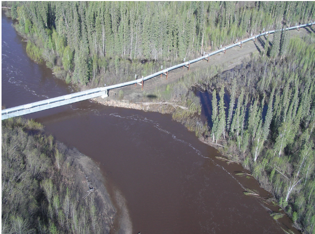
Figure 1. Hess Creek looking downstream, spring 2005 breakup. Hydraulic and thermal erosion of right bank resulting in misalignment with pipeline bridge.
