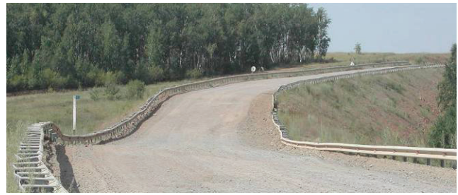
Figure 8. A section of road on the “Amur”–Chita to Khabarovsk Highway, km 247, before repairs, July 2006.
