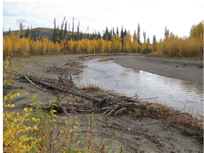
Figure 6. Looking upstream from the bridge, September 2007, showing scallops between deflector vanes and woody material that accumulated along the bank and floodplain.
