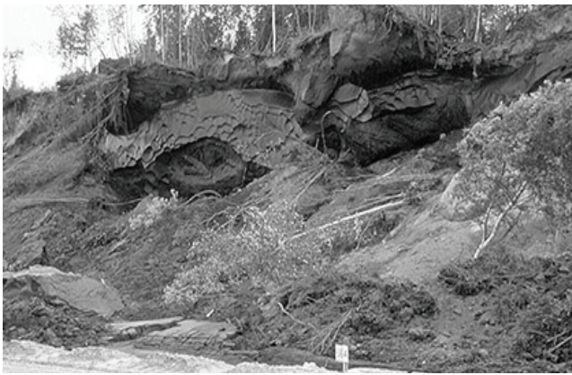
Figure 2. Thaw degradation of cutslope in ice-rich permafrost inducing slope failure (ADOT&PF file photo).
