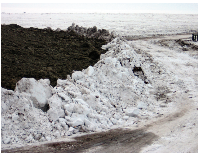
(7c) Close-up view of newly-placed snow berm and ice-rich permafrost waste material behind snow berm.
