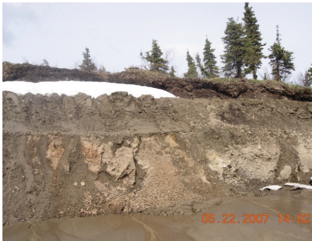
(5b) Advanced thaw condition along ice-rich permafrost cutslope shows ditch filling with saturated silt.
