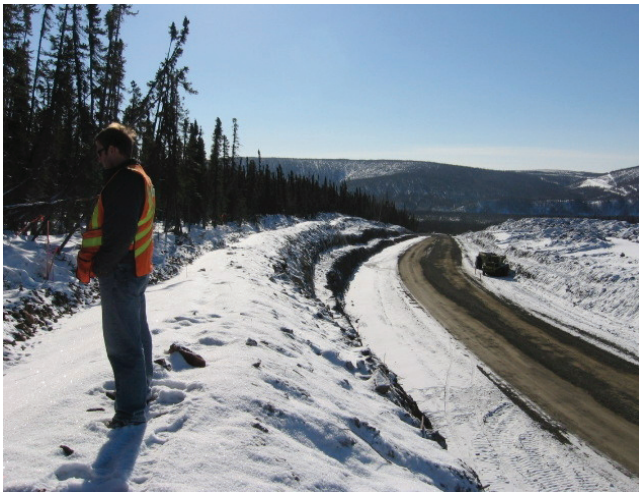
(4a) Newly-constructed cutslope in ice-rich permafrost. Note interceptor ditch at slope top and stepped cut face.
