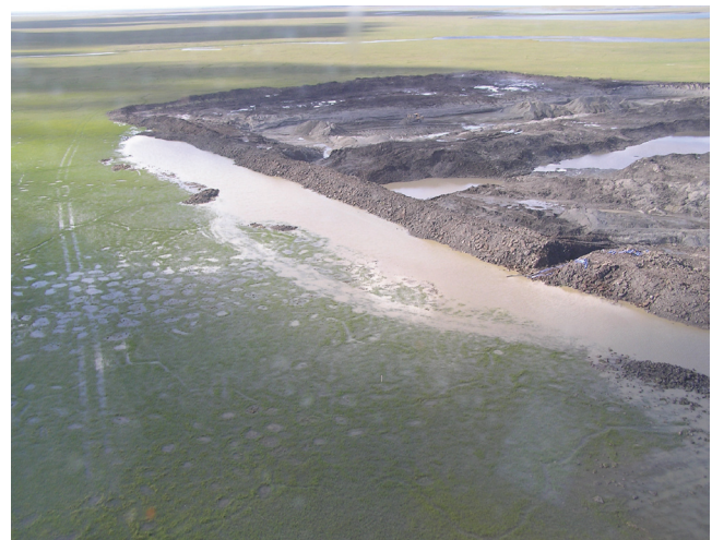
Figure 6. Containment structure for excavated permafrost on the North Slope of Alaska (photograph courtesy of G. Griffin).
