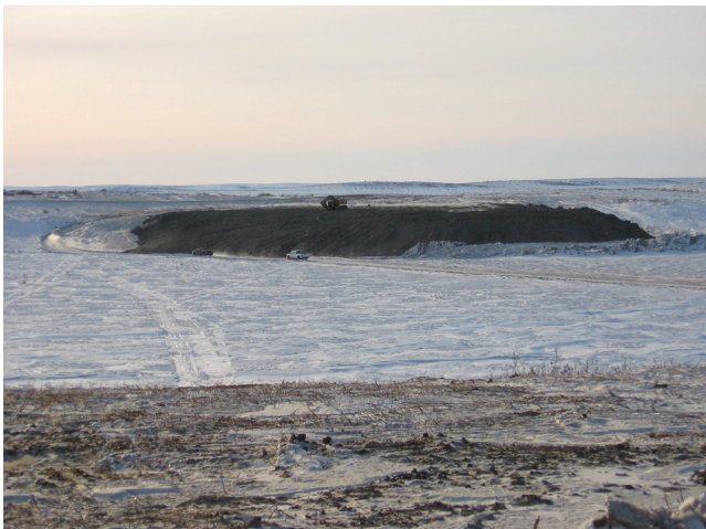
(7b) Snow berm surrounding right side of ice-rich permafrost waste pile (shown in upper right of photograph [7a]).
