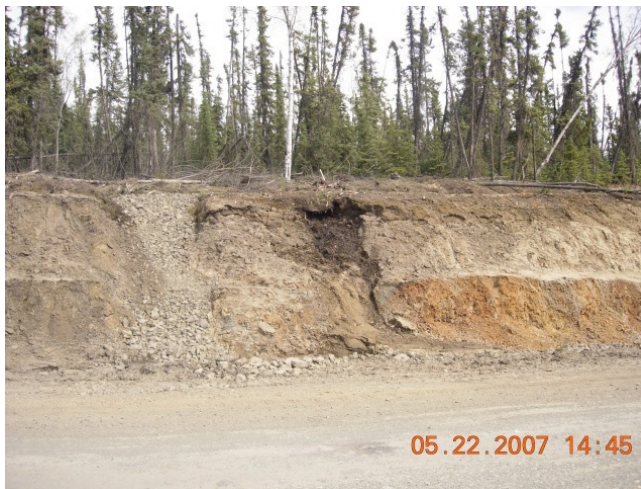
(5a) Pockets of thaw failure along cut face. —A gravel drainage blanket (left side of photo) was installed to slow thawing, retard slumping of thawed material, and provide drainage during the thawing process.
