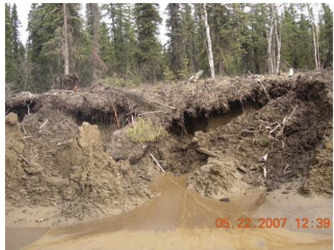
(5c) Advanced thaw degradation of cutslope shows block failures and runoff of highly fluid silt into ditch.
