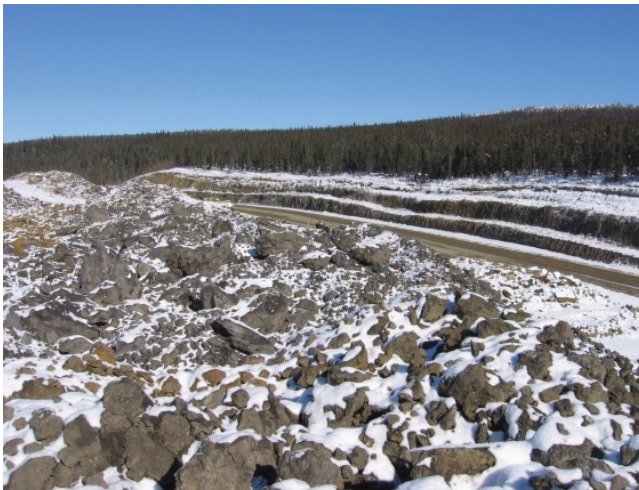
(4b) View across permafrost waste pile at newly cutslope face in ice-rich permafrost. The volume of waste exceeded the boundary limits of the permitted area.
