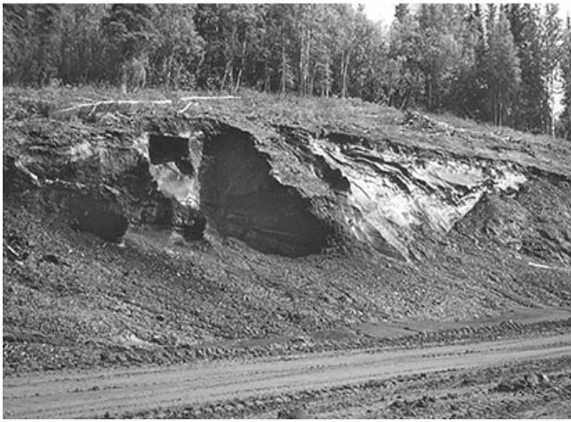
Figure 1. Road cut in ice-rich permafrost (ADOT&PF file photo).
