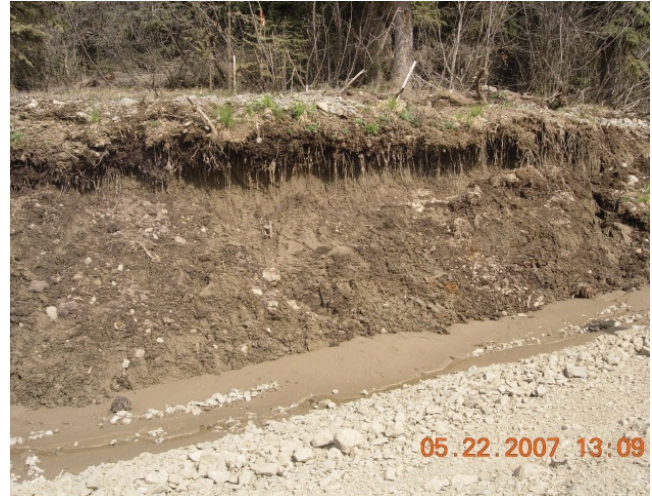
(5d) Advanced cutslope thaw with silty runoff flowing in ditch and general slumping of coarser material.
