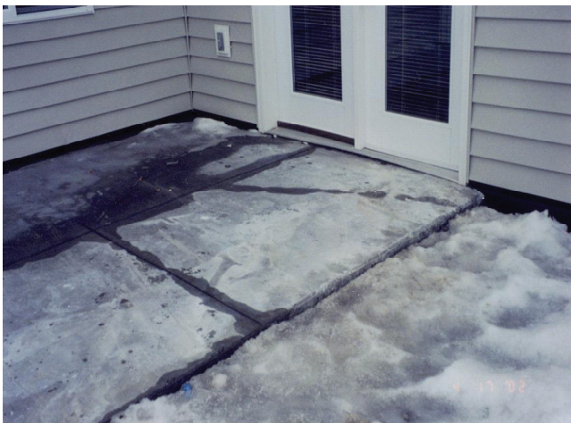
Figure 4. Uplifted concrete patio slab. Door sill and jambs were lifted by patio slab.
