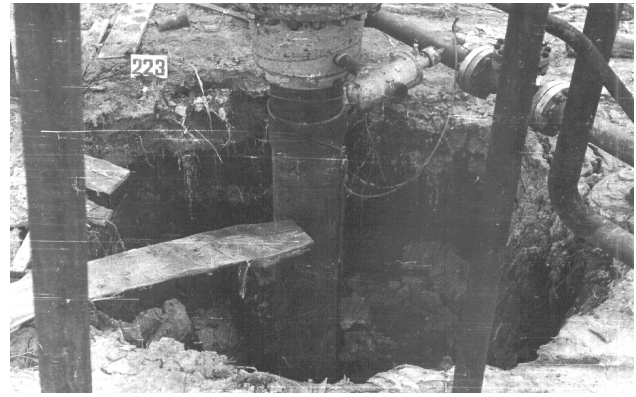
Figure 4. The thermokarst funnel around production wellhead.
