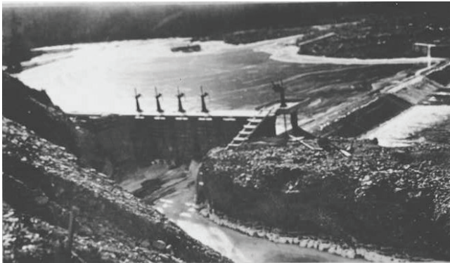
Figure 4. Intake and diversion dam at headwaters of Chatanika River.
