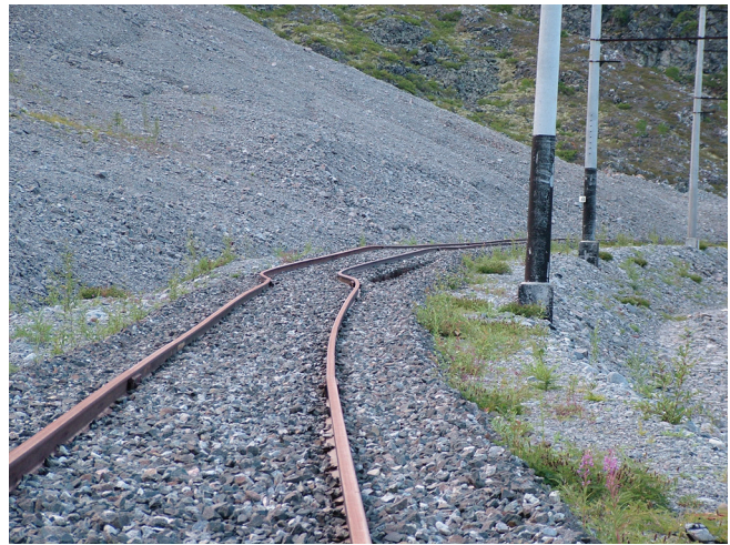
Figure 7. Deformations of the railroad bed (Chara-Cheena).
