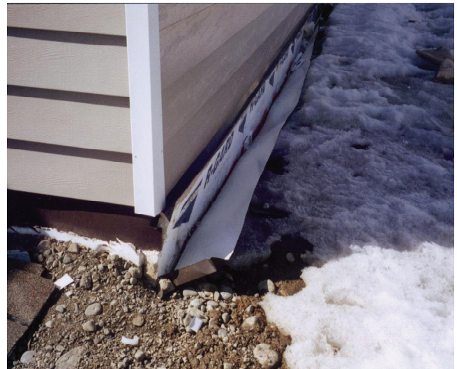
Figure 5a. Displaced vertical insulation board with flashing partially removed.
