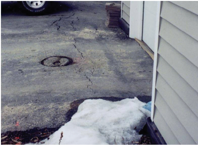
Figure 3b. Garage door and driveway entry with pavement fracture above outside edge of buried horizontal insulation board. Note temporary tapered wood spacer between uplifted asphalt pavement and garage door.
