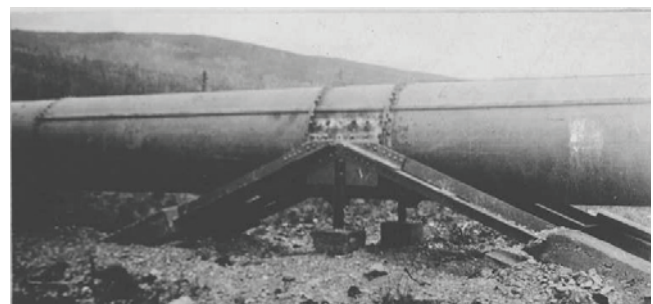
Figure 5. Typical siphon pipe anchor.
