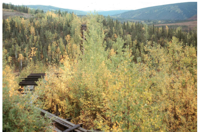
Figure 13. Wood outlet structure at siphon valley crossing, fall, 1970.
