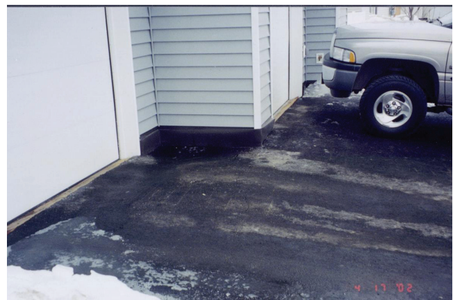
Figure 3a. Ponded water against building between driveway in insulated area that did not heave.
