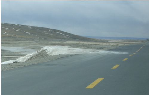
Figure 11. Icing and frost mound along the QHT.
