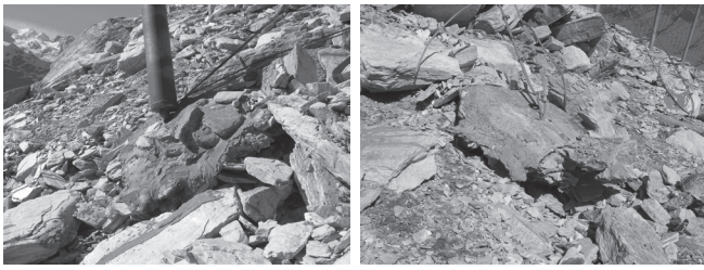
Figure 9a. Dislocated swivel support (left). Fig. 9b. Tipped concrete foundation (right) in the damaged snow net rows 5 and 6.
