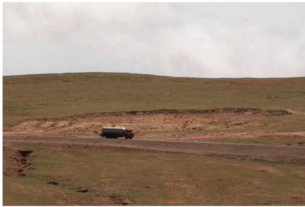
Figure 2. Thaw slumping at K3035 mileage of QTH.
