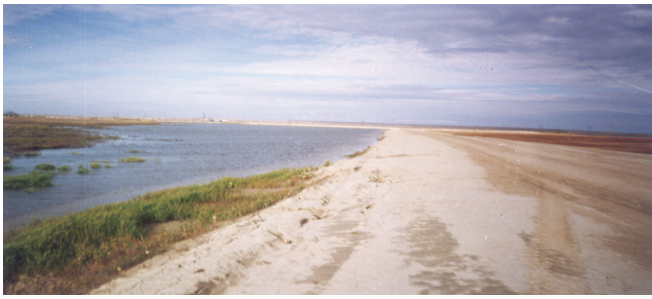
Figure 3. Impoundment of the road surroundings, northwestern Siberia.
