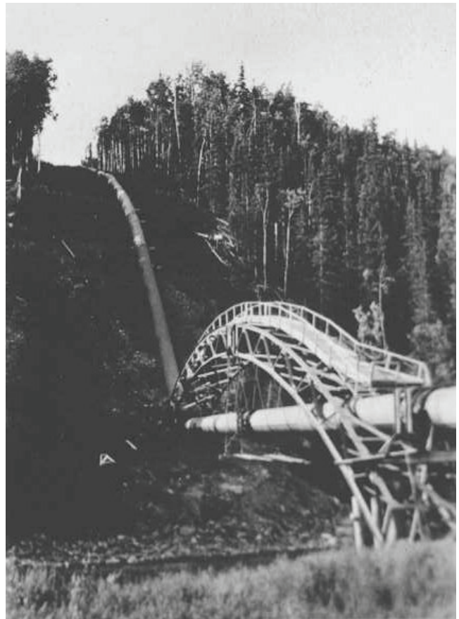
Figure 8. Chatanika River siphon and steel arch bridge crossing.
