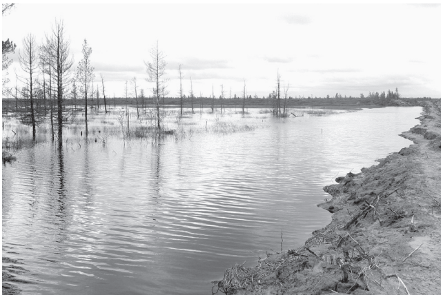
Figure 10. Flooding of the area adjacent to the pipeline in the vicinity of transect I-I. View from the gas pipeline.
