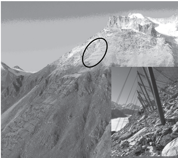
Figure 1. The study site Wisse Schijen with 8 rows of snow nets is located in the upper part of the slope (outlined). Row 2 is shown inset. Several rows of snow bridges are visible in the slope sector below.
