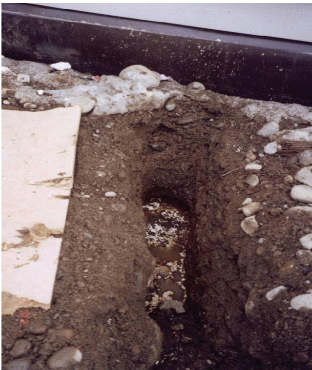
Figure 6. Test pit exposing horizontal insulation board. Air gap was found between insulation board and overlying frozen soil that was lifted by adjacent deeper frozen ground.
