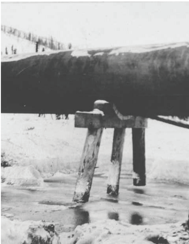
Figure 6. Typical siphon pipe support on timber pile trestle bent.
