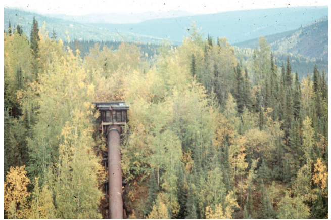
Figure 12. Inlet structure and siphon pipe, fall, 1970.
