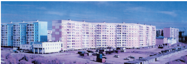
Figure 1. Housing estate erected in Yakutsk on back-filled ground.
