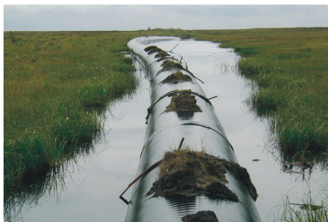
Figure 5. Deformations of the pipes due to thermokarst subsidence and frost heave processes.
