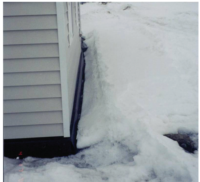
Figure 5b. View of perimeter base flashing covering vertical insulation board. Flashing has been slightly distorted by upward board movement.
