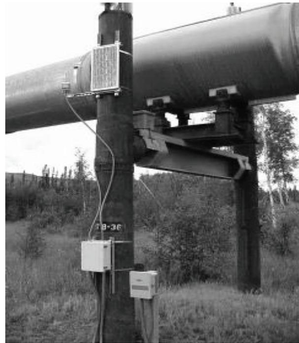
Figure 2. Installation of photovoltaic panel, battery box, data logger enclosure on VSM and thermistor string enclosure.
