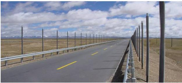
Figure 4. Thermosyphone installed along the QTH to treat thawing settlement.
