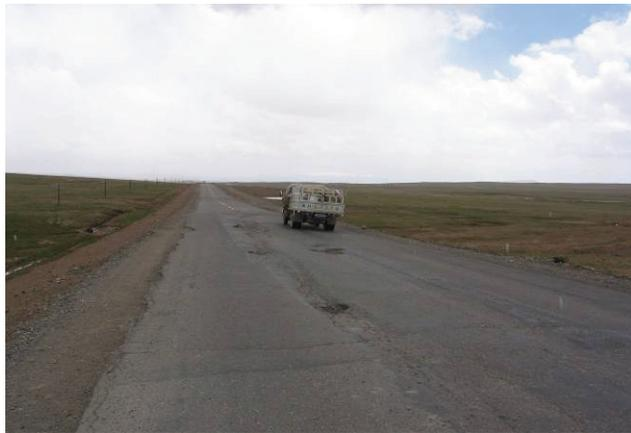
Figure 2. Longitudinal cracks and settlement developed in the embankment of the QTH.
