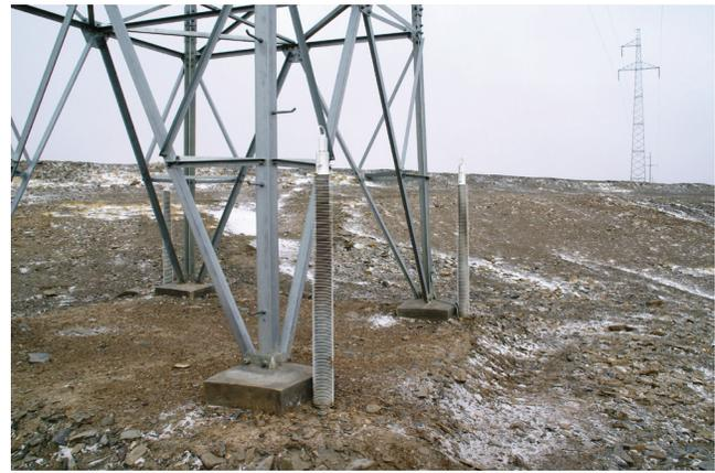
Figure 7. Enlarged picture for details of the thermosyphon-cooled tower foundation.
