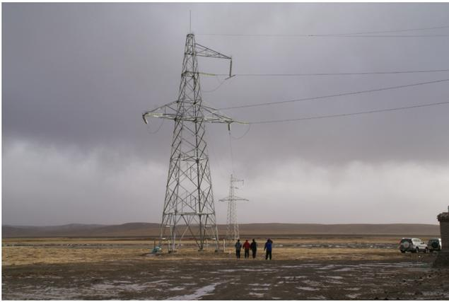
Figure 6. Thermosyphon-cooled tower of power transmission line in alpine meadow in the vicinity of Damxung along the Qinghai-Tibet Highway. The thermosyphons were installed in each of the four feet of the tower supported by mat/pile foundation.
