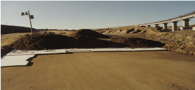
Figure 5. Insulation layer installed along the QTH to keep the underlying permafrost.
