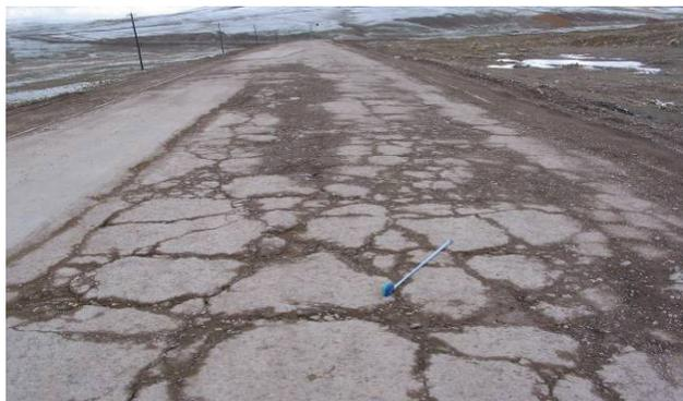
Figure 3. Crack damage of the concrete surface layer.
